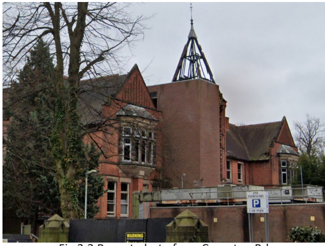
Fig 2.2 Recent photo from Compton Rd.
